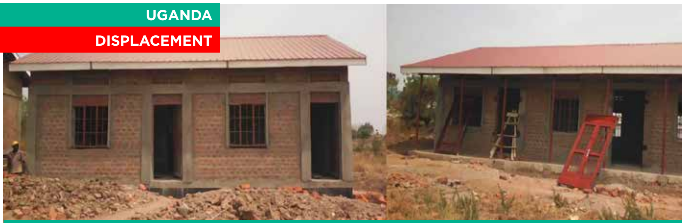
A newly constructed teacher's residence and an administration block at Ariwa Primary School. Photo by CRS staff
